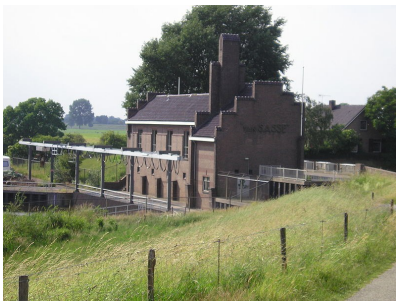
Pumping station elevating the drainage water for evacuation
