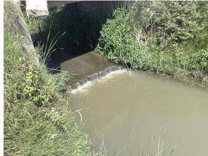
Open collector drain
