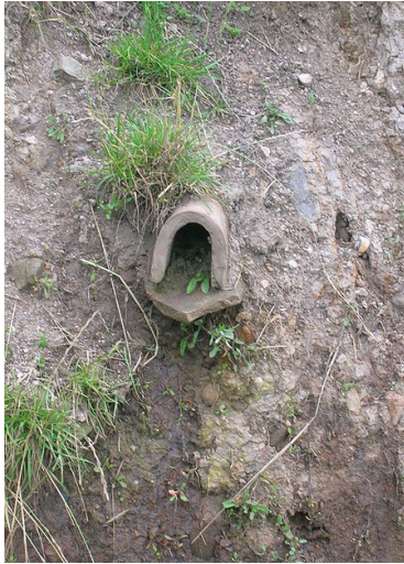
Outlet of an old tile drain
