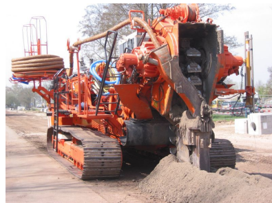
Drainage machine burrying plastic drainpipes.
