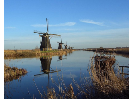
Antique windmilss evacuating the drainage water from the interior polders to the river between levees
