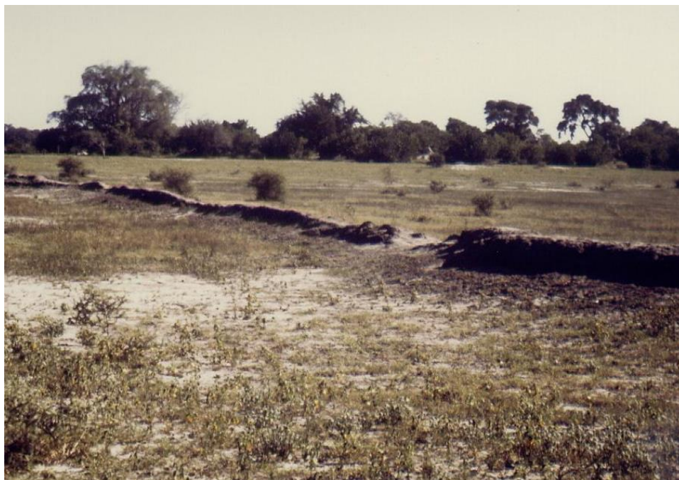
Old, abandoned traditional bund made to retain water in the molapo for flood-recession cropping
