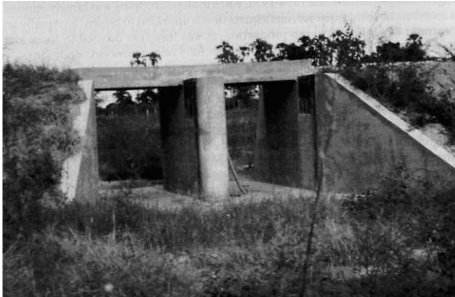
Photo 6. Close up of the sluice gate of the bund in Photo 5.
