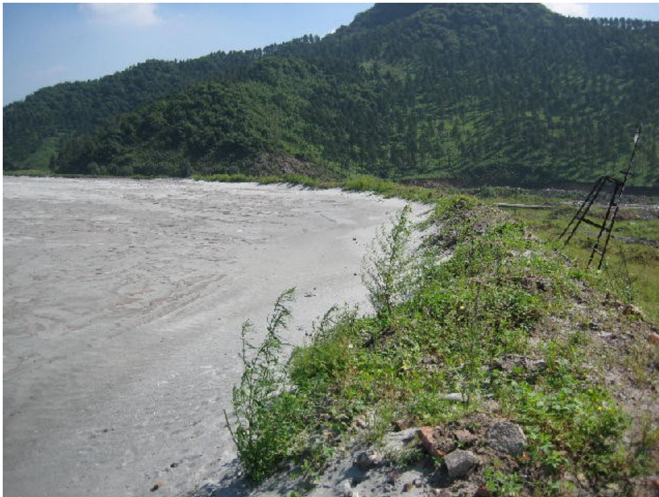
Top of the dam containing the tailings deposit that can be seen to the left.
