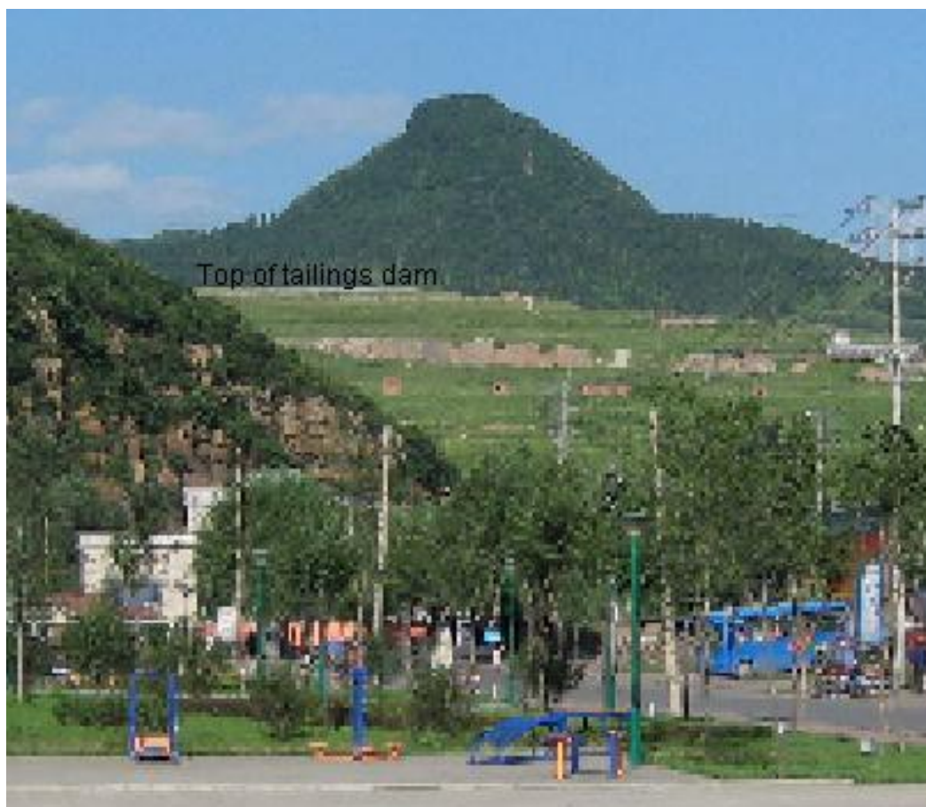
The top of the dam containing the tailings deposit seen from Nanfen city
