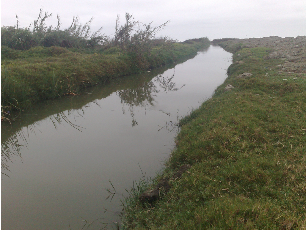
Photo 3. In the lower reaches of the central drain the water level is too high to permit properly functioning lateral drainage systems. A pumping station is required.
