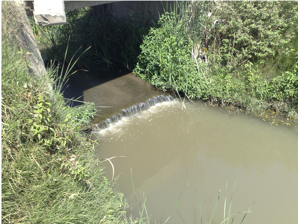
Photo 1. The recently cleaned central drain is discharging about 10 l/s.
