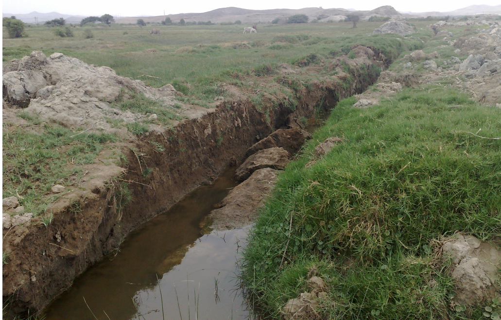
Photo 2. The recently excavated lateral drain collapses due to steep side slopes.
