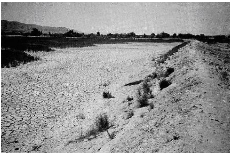
Photo 1. Earthen bund for water harvesting
