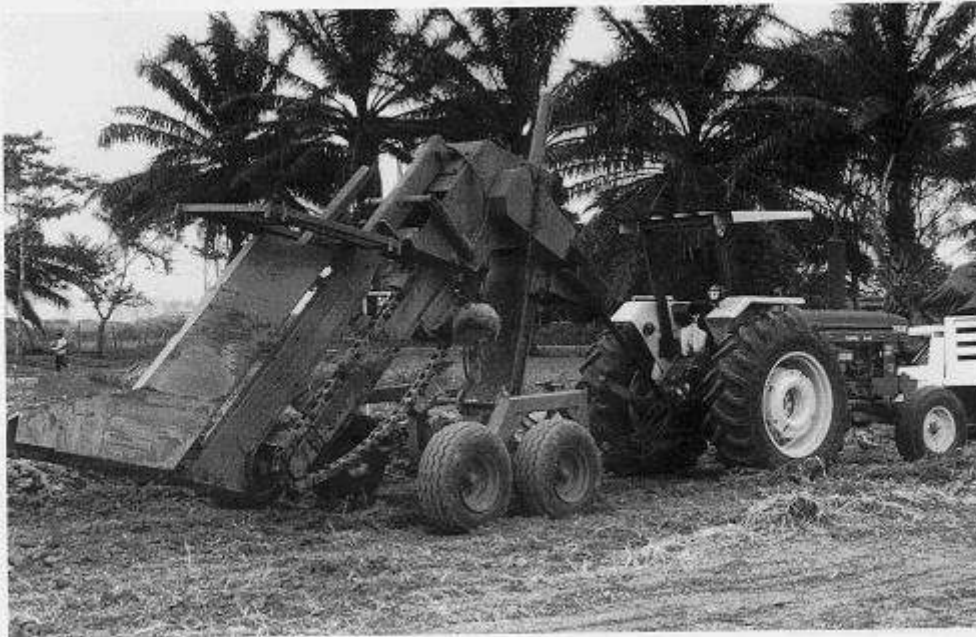
Photo 2 Tractor-drawn drainage machine with chain box
